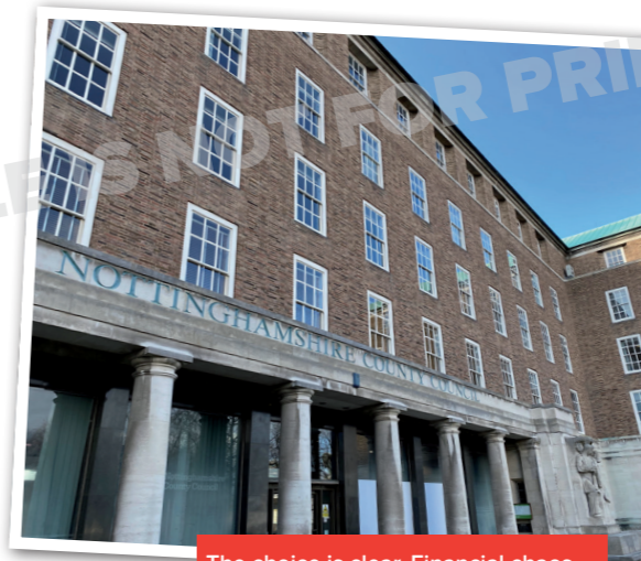
The choice is clear. Financial chaos under Labour. Or a high quality, value for money Conservative-led council.
